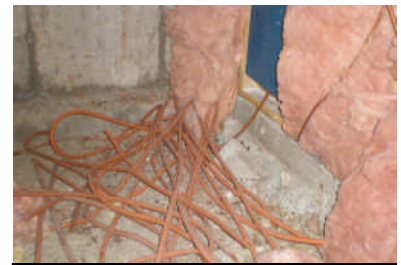
Old Entran tubing on ground in crawls
